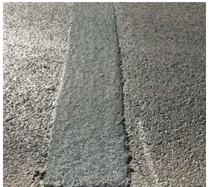
In-house manufactured Roadflex applied as part of the works
