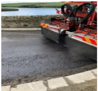
Multibond 70 emulsion coat & Fortifix bond before overlay
