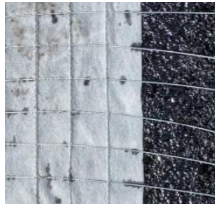
Multibond 70 emulsion coat & Fortifix bond before overlay
